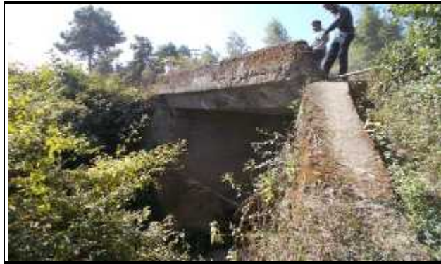
RCC Slab Bridge
