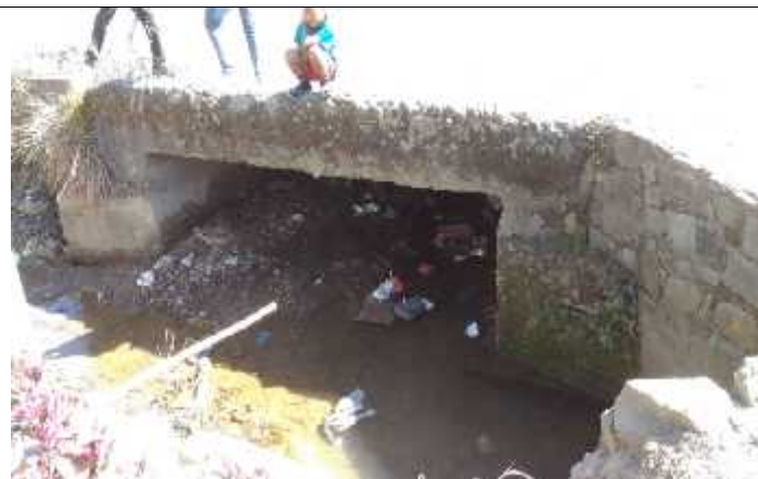
Slab Culvert (Ch. 4.061 Km)
