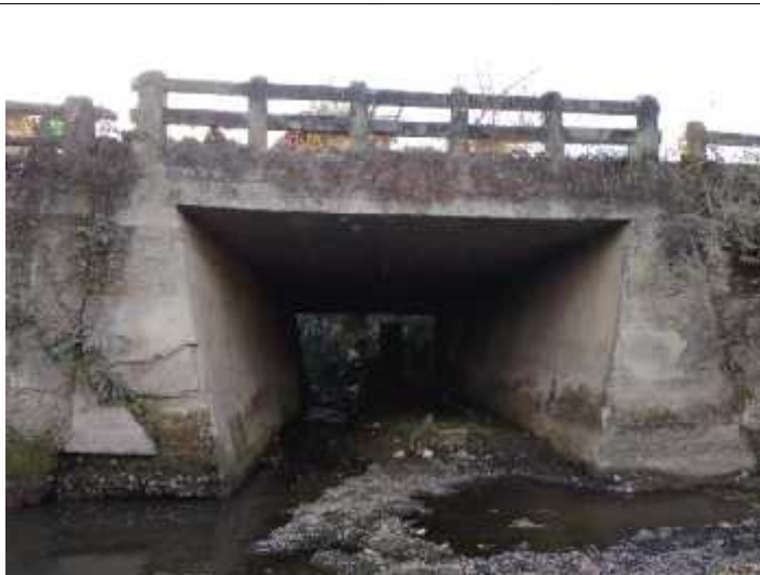
RCC Slab Bridge (Ch. 2.380 Km)
