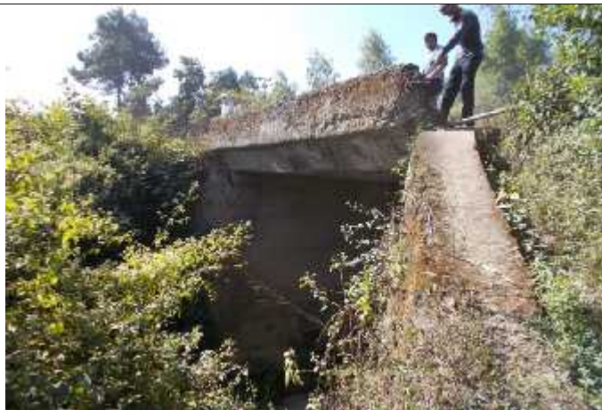
RCC Slab Bridge (Ch. 13.557 Km)
