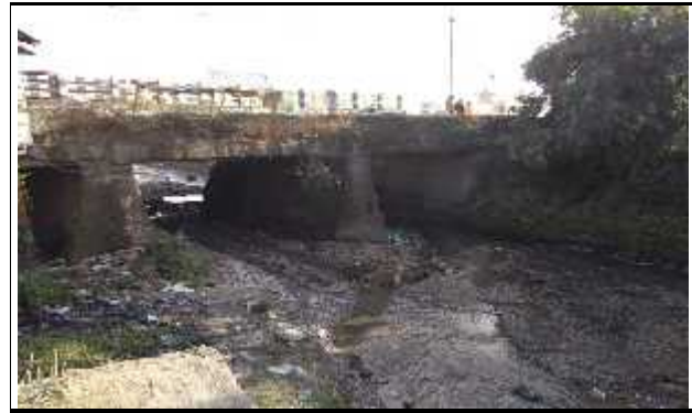
RCC Slab Bridge
